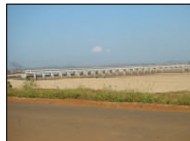
View of Naraj barrage in dry season
